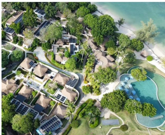
Solar Rooftop at The Naka Island, a Luxury Collection Resort and Spa, Phuket Thailand
