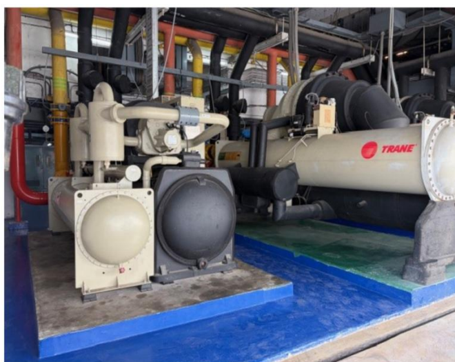
Right: Upgrading Chiller Plant System at JW Marriott Bangkok
