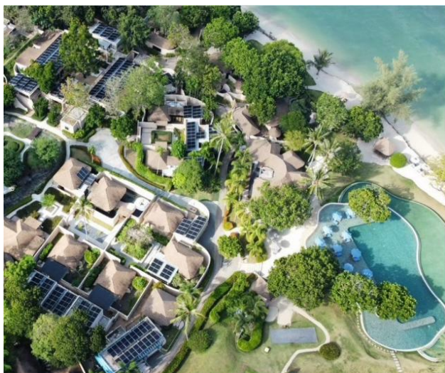
Left: Installation of Solar Rooftop at the Naka, a luxury resort and spa, Phuket
